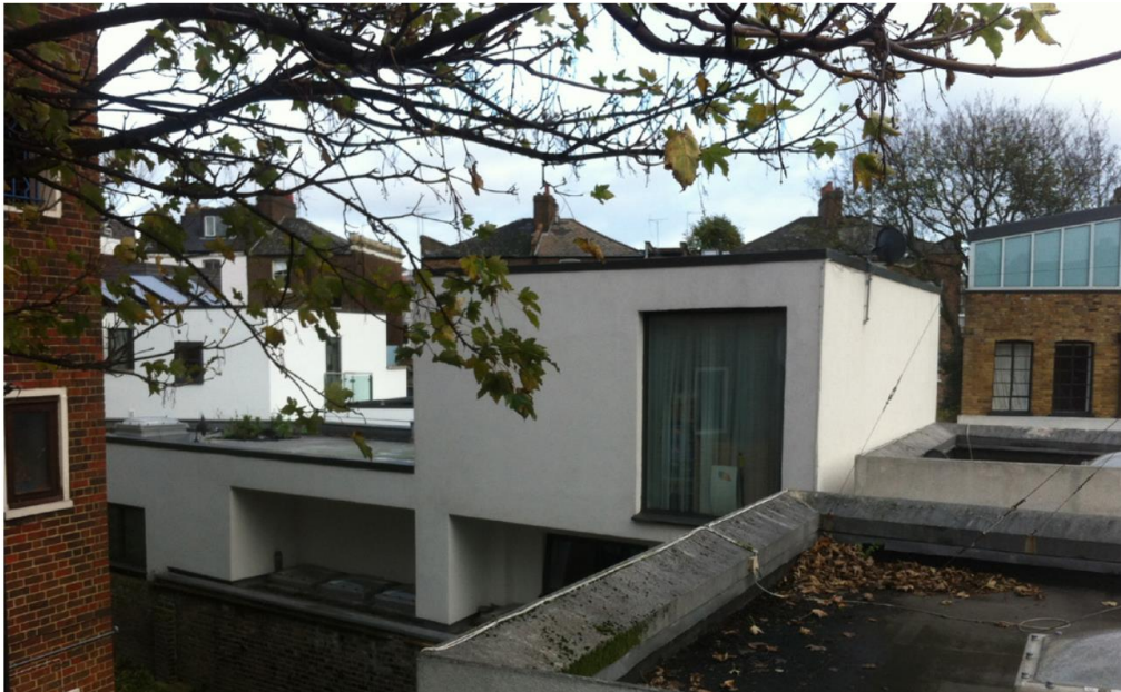
Image 6. – View towards first and second floor windows of 37L Mildmay Grove North from flat roof of 4 Colony Mews
