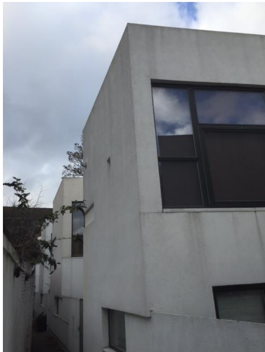
Image 5 – View from access path towards site
