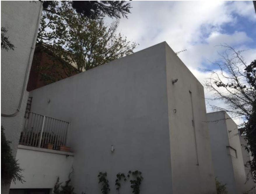
Image 4. – View of existing flat roof from west of site
