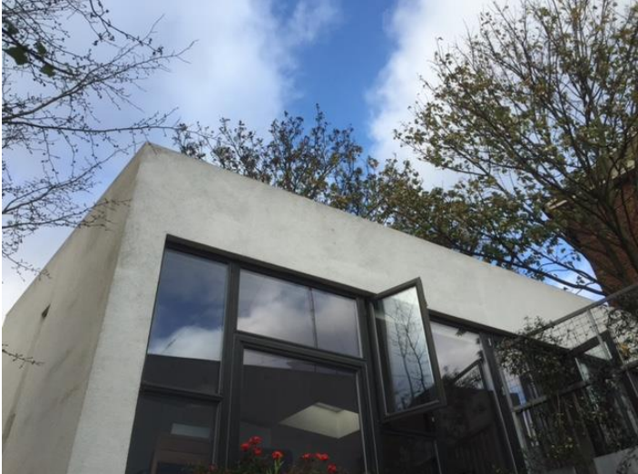
Image 3. – View of existing flat roof from east of site
